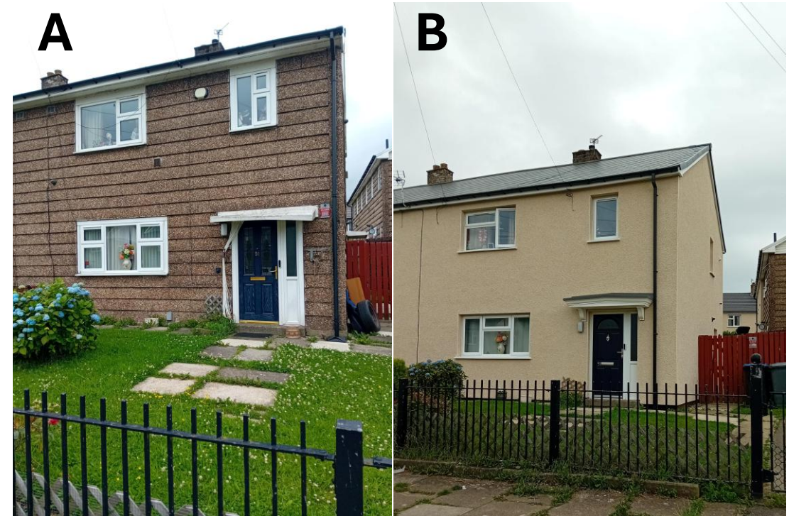
Before (A) and after (B) illustration of external wall retrofitting with a white render finish, applied on top of thermal insulation boards. Image credit: Incommunities
