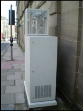
City monitoring station
